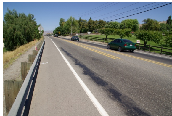
FIGURE 10 Typical views of SR 28 before the project showing substantial wheelpath cracking and flushing.
