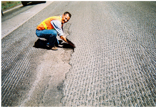
FIGURE 33: Milled surface of SR 97A showing de-bonded area.
