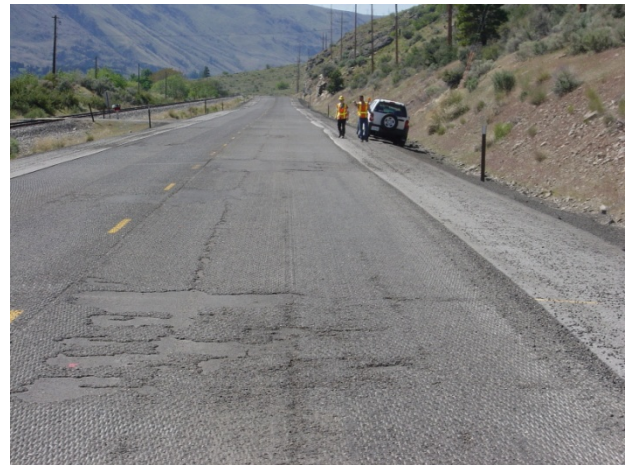
FIGURE 34: Milled surface of SR 97A showing de-bonded area probably from construction-related temperature differentials and gear box streaking.
