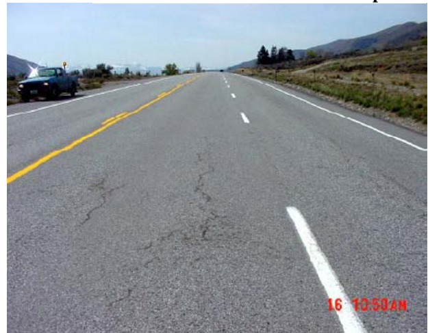
FIGURE 31: Looking south from MP 207.37 showing wheelpath cracking.
