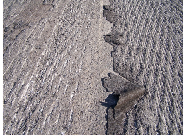
FIGURE 18: Milled surface of SR 28 showing fabric.
