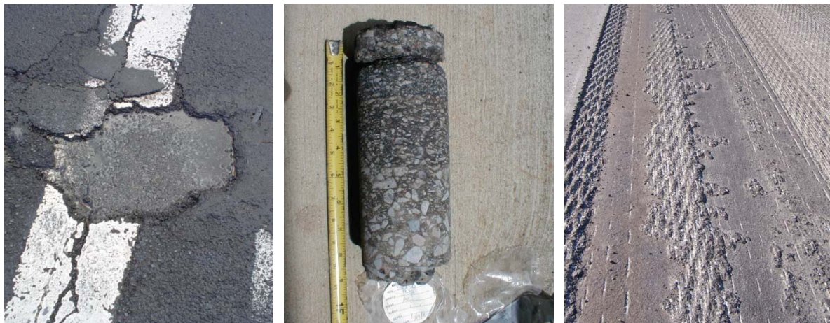
Figure 1: Three types of evidence for de-bonding: shallow potholes (left), detached cores (middle) and loosely attached pavement after milling (right).
