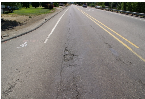
FIGURE 10 Typical views of SR 28 before the project showing substantial wheelpath cracking and flushing.
