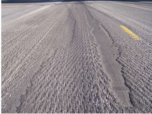
FIGURE 17: Milled surface of SR 28.
