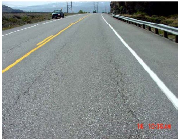
FIGURE 30: Looking south from MP 202.50 showing wheelpath longitudinal cracking.
