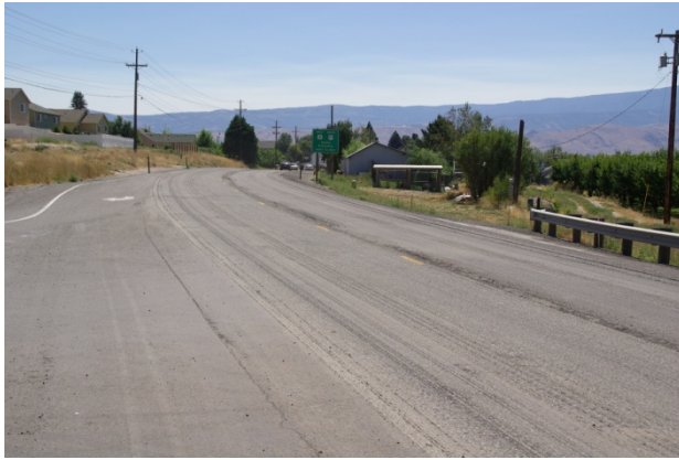
FIGURE 15: Milled surface of SR 2/97.
