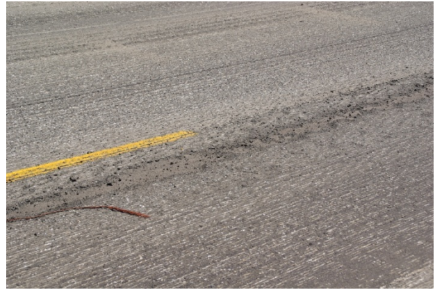
FIGURE 16: Milled longitudinal joint area.
