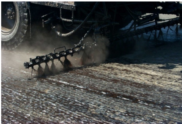
Clogged nozzles on SR 500
